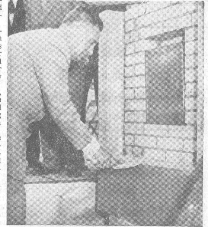
CORNERSTONE LAYING. A. L. (Dutch) Schwab of New Philadelphia, a member of the Union Hospital board of trustees, did the official honors in 1951 when the cornerstone was laid for the addition to Union Hospital.
